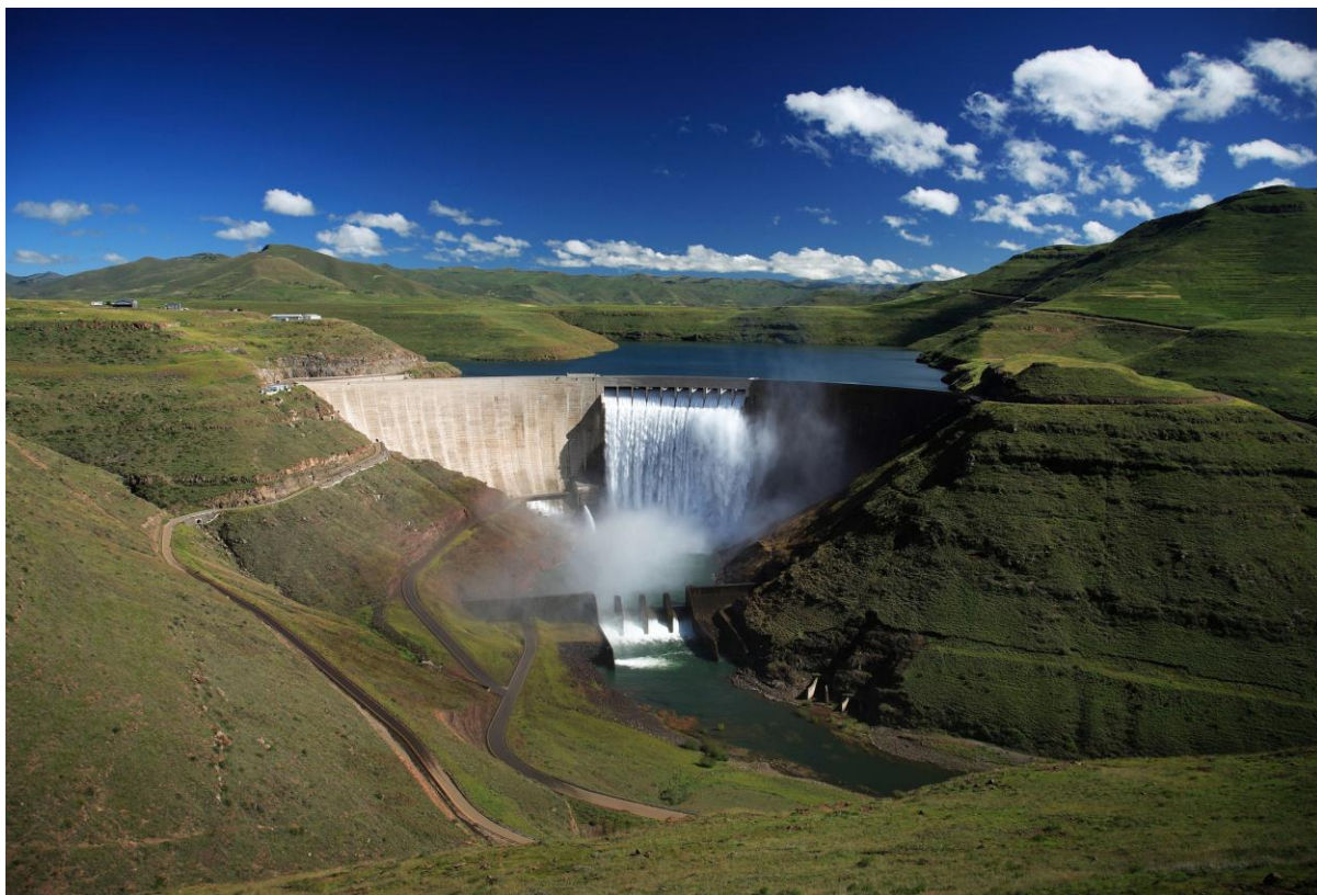
The Katse dam wall, Lesotho Highlands Water Project. Source: Adobe
